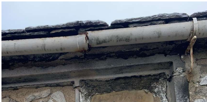
photo 14 – open gutter joint to tower
