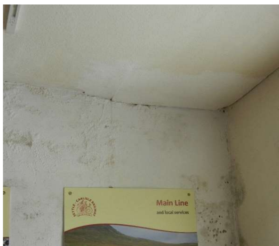
photo 29 – SE corner gallery R202
