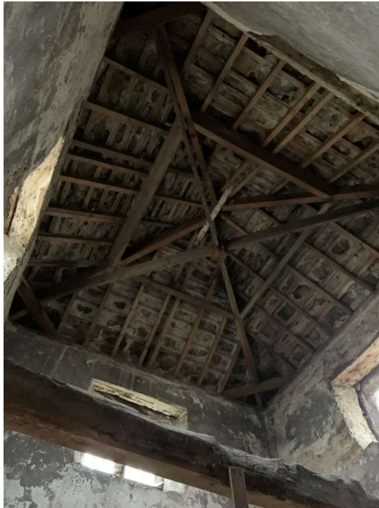
photo 10 – tower roof structure
