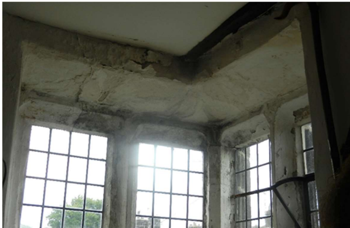
photo 30 – window head W112/113
