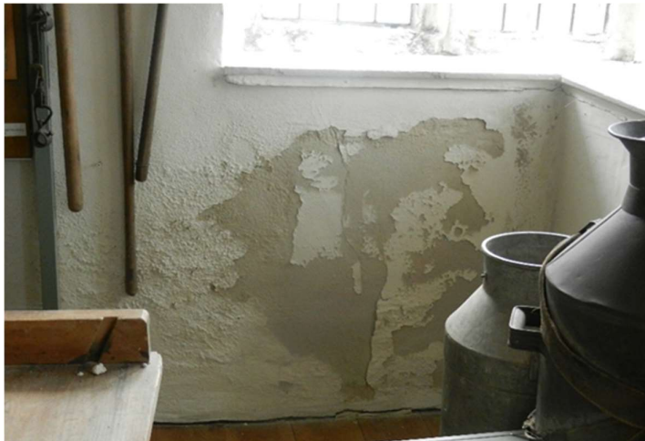
photo 31 – wall below W113
