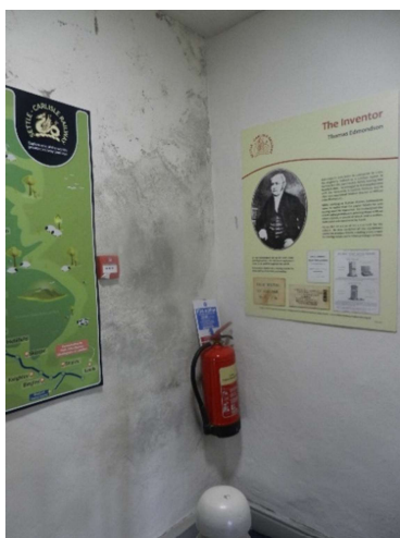
photo 28 – 2 nd floor SW corner rear stair
