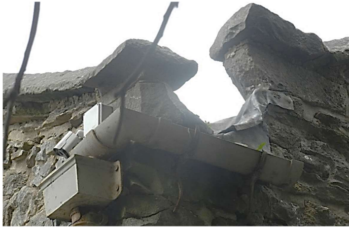
photo 6 – rainwater outlet from valley gutter over SW corner of rear staircase
