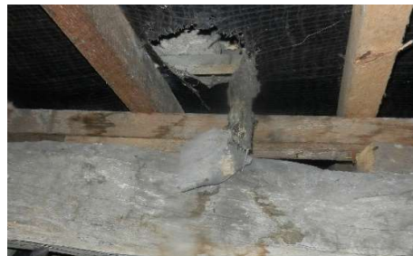
photo 9 – roof over R207
