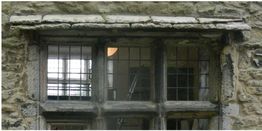
photo 20 – Window head W115
