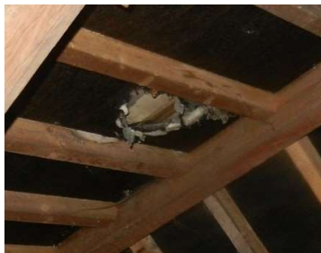
photo 8 - roof over R202
