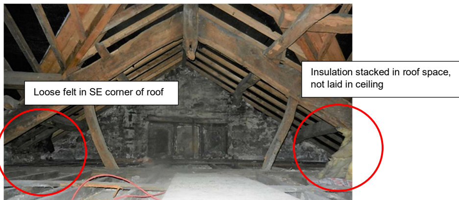
photo 7 – roof space over gallery R202
