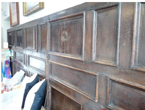
Fig,21: re-set panelling to south wall
