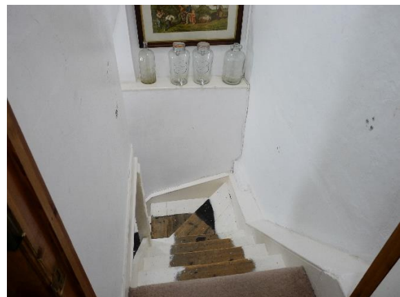
Fig.67: 19 th century staircase, from the east
