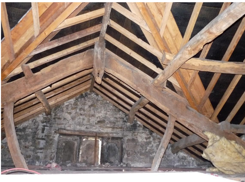
Fig.72: south wing roof from the east
