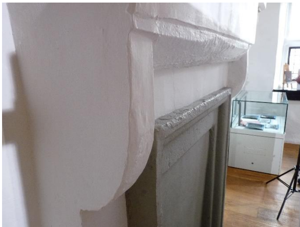
Fig.36: hall chamber fireplace
