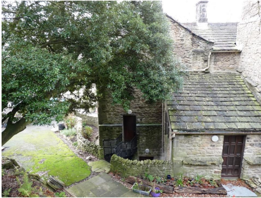
Fig.8: south-east outrigger and east gable of south wing, from the east
