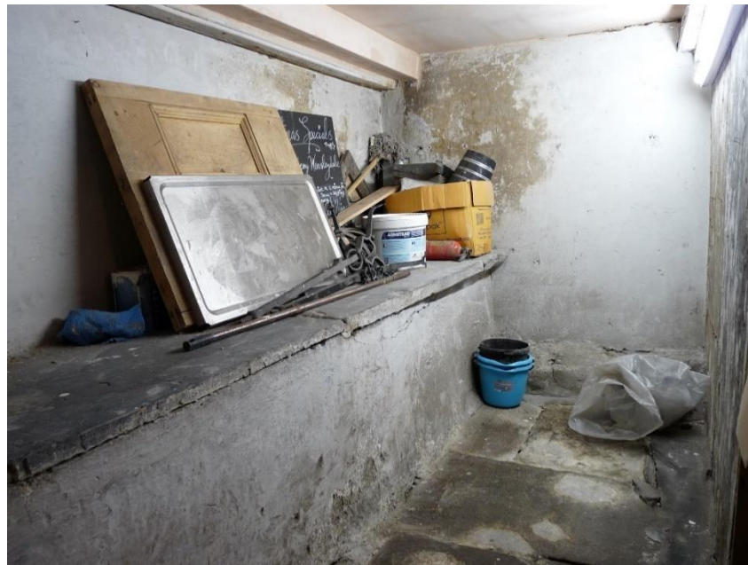
Fig.25: 'cellar' below the staircase
