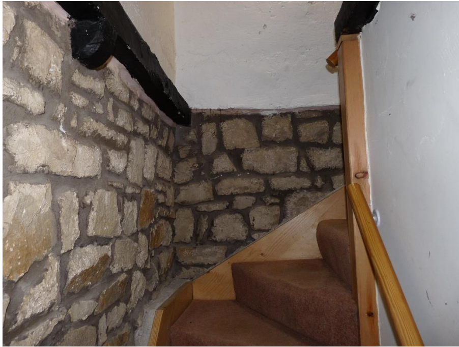
Fig.28: staircase from the south
