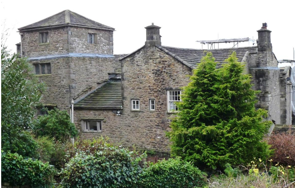
Fig.7: Rear of the tower, north-east outrigger and north wing from the north-east
