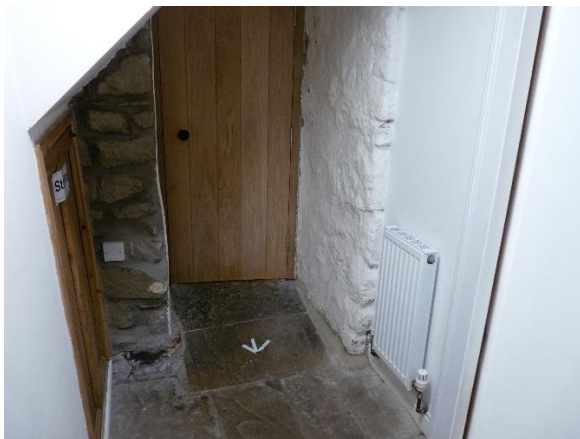
Fig.26: lobby and door into G12, from the south
