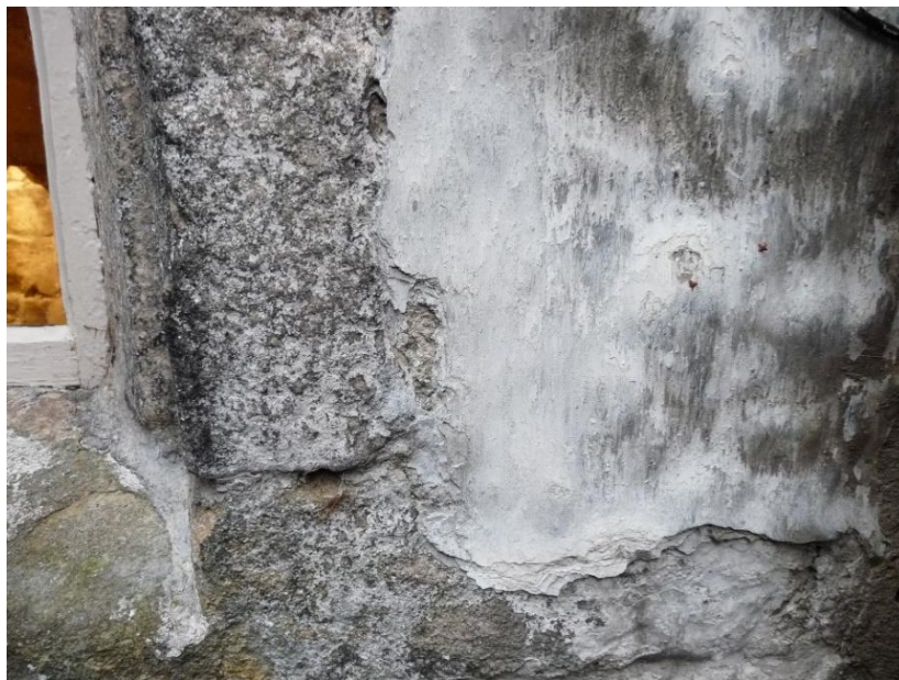
Fig.15: layers of lime wash on the north elevation
