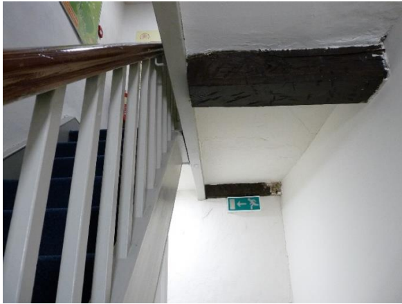
Fig.39: truncated beams for staircase
