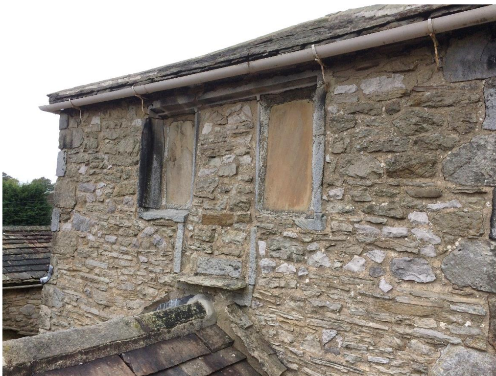
Fig.75: west face of the tower, from the roof, with central 'doorway' to the blocked window (photo: Lynn Northrop, Overton Architects)
