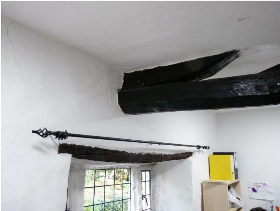
Fig.65: window and east end of half-truss, from the north-west
