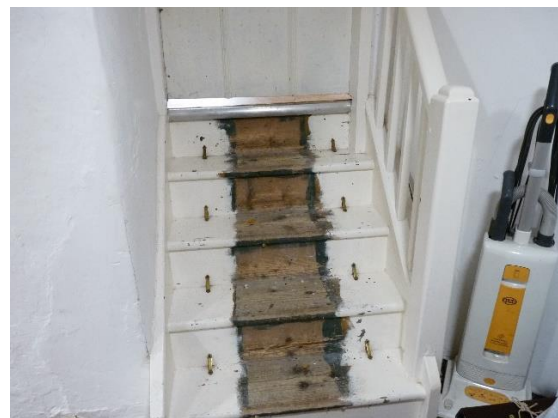
Fig.48: stairs up to F9, from the landing
