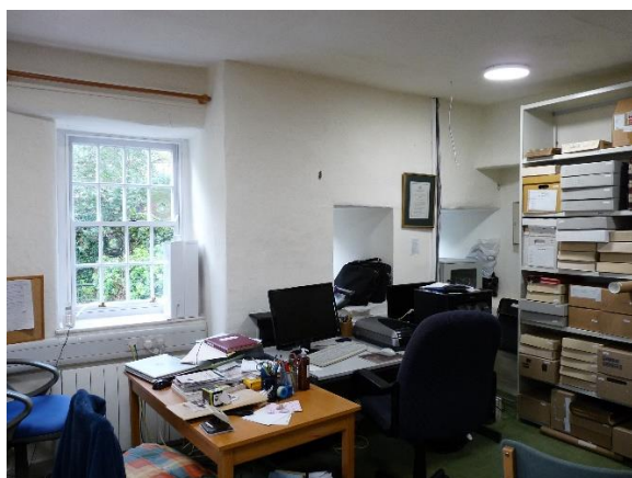
Fig.63: altered east wall with former doorway to left
