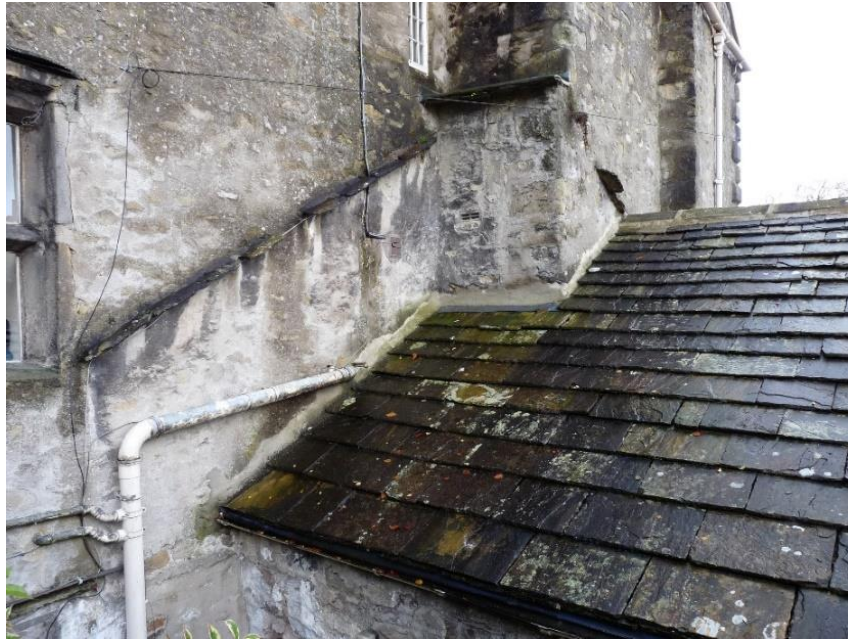
Fig.12: tabling to an earlier and higher roofline on the north elevation
