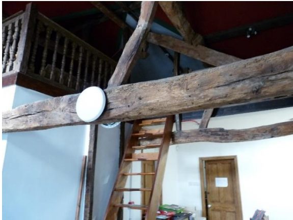
Fig.58: roof trusses and ladder, from SW
