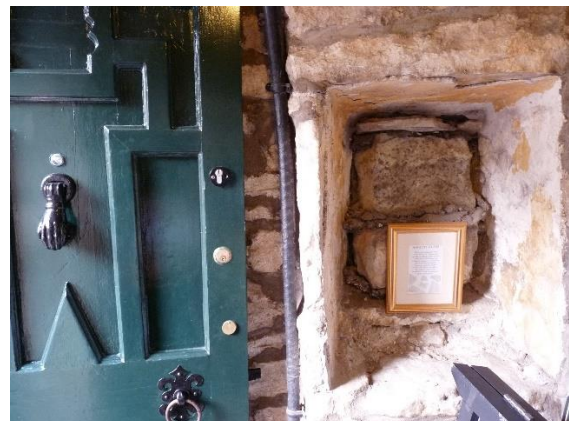
Fig.31: outer door and blocked north window
