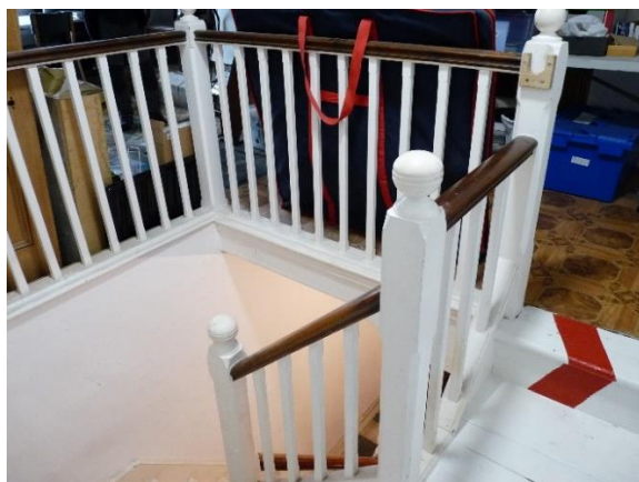
Fig.56: top of staircase, from south-east
