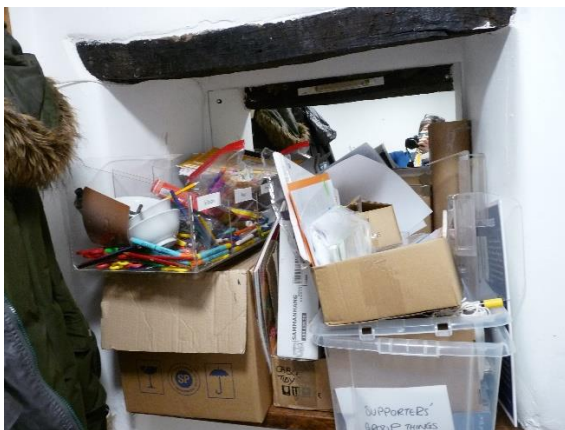
Fig.66: blocked opening on north wall
