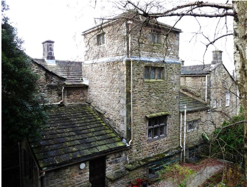
Fig.13: rear elevation with stair tower and plainer windows, from the south-east
