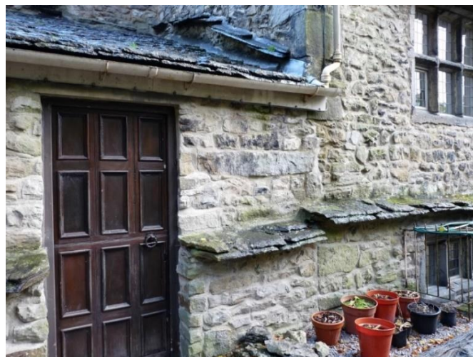
Fig.14: tabling and the masonry joint between the stair tower and south-east outrigger. The doorway is an insertion
