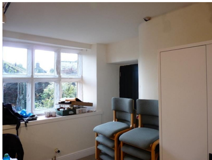
Fig.46: east room in north wing, from the south
