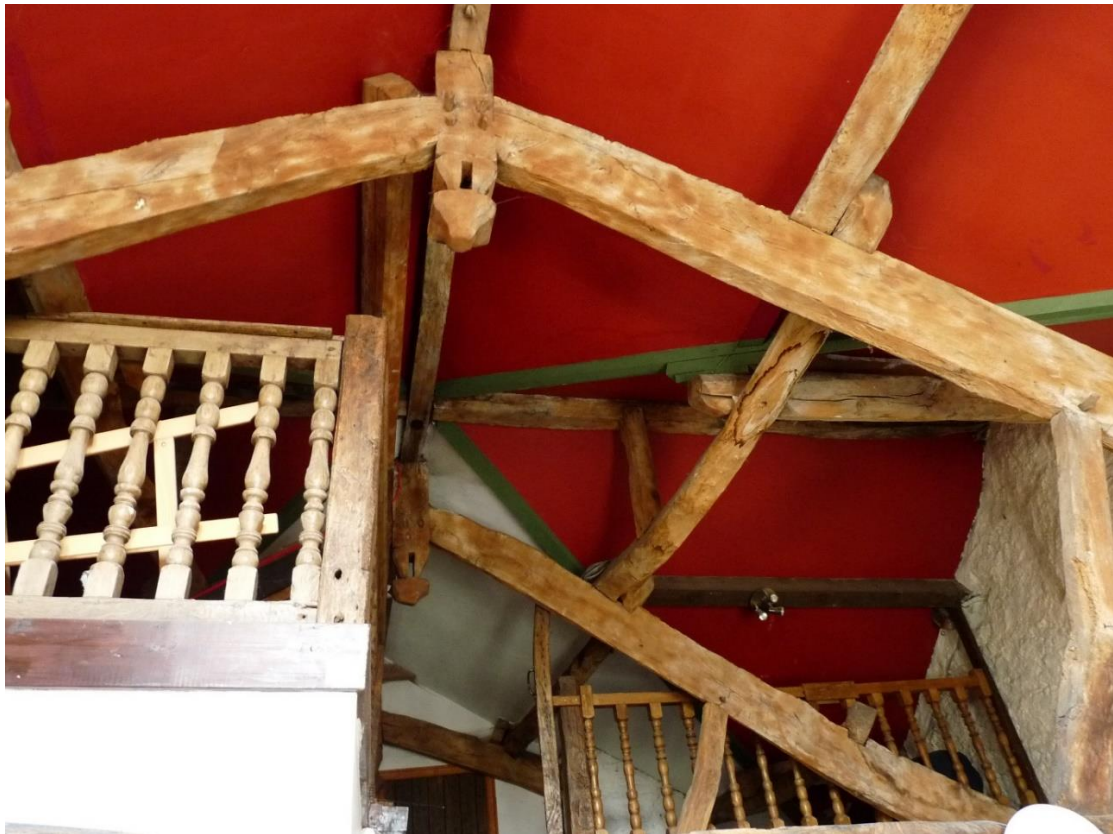
Fig.68: king-block roof trusses in the north wing, from the west
