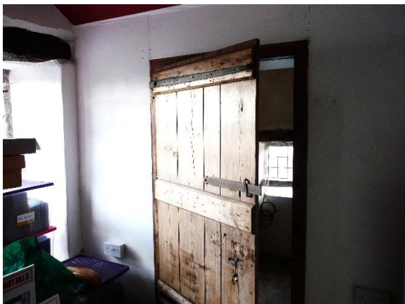
Fig.60: doorway to closet from S6
