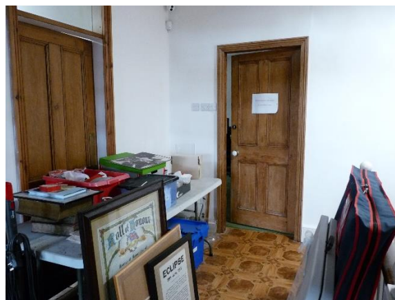
Fig.57: doors to S8 and S9, from west
