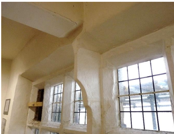
Fig.52: stone king mullion corbel to tie-beam
