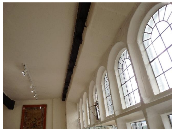
Fig,22: hall window and sleeper beam
