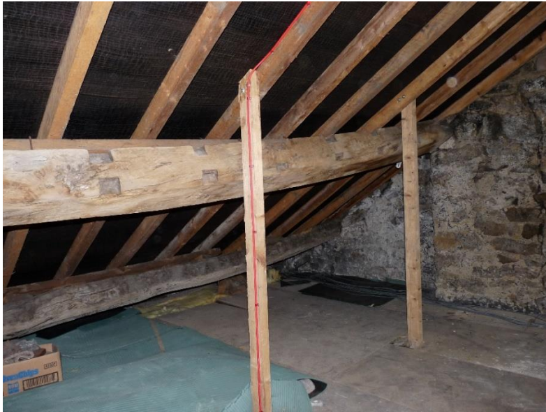
Fig.69: north bay of north wing roof, with re-used floor beam for a purlin
