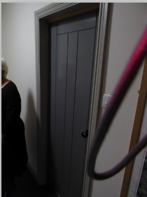
Plate 20. Modern door to be replaced
