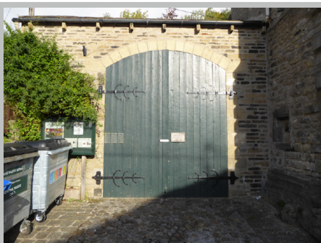
Plate 5. Garage/coach house doors
