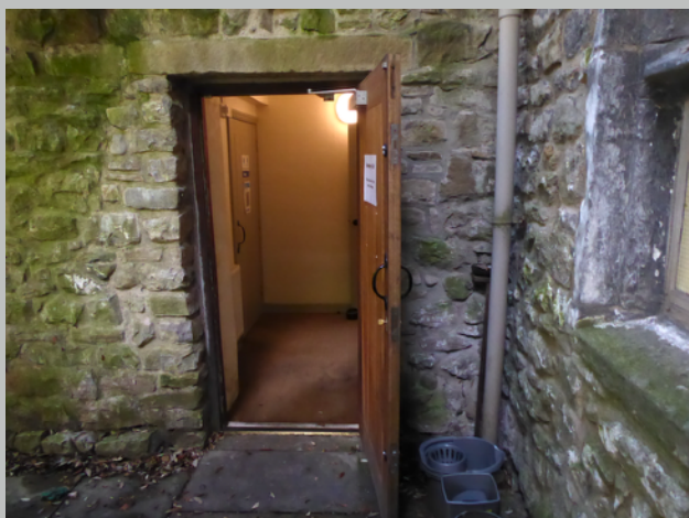
Plate 17. Doorway to be widened
