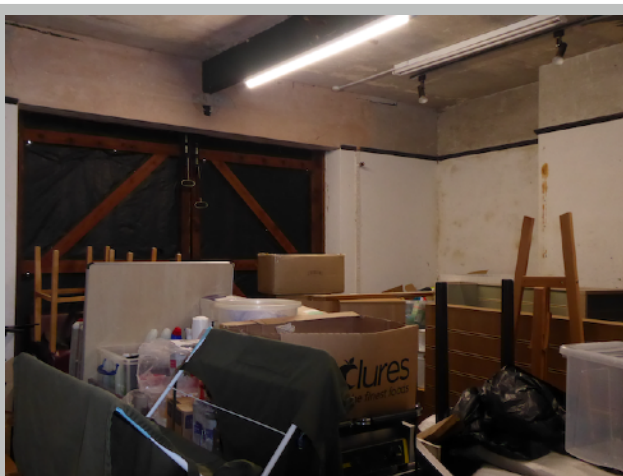
Plate 6. Interior of garage/coach house doors
