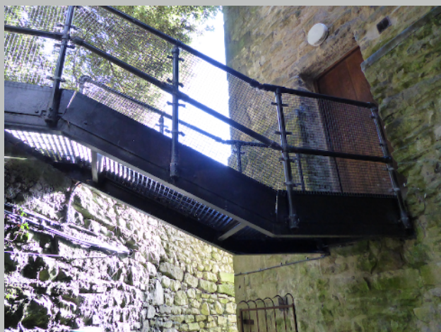
Plate 18. Bridge to be removed
