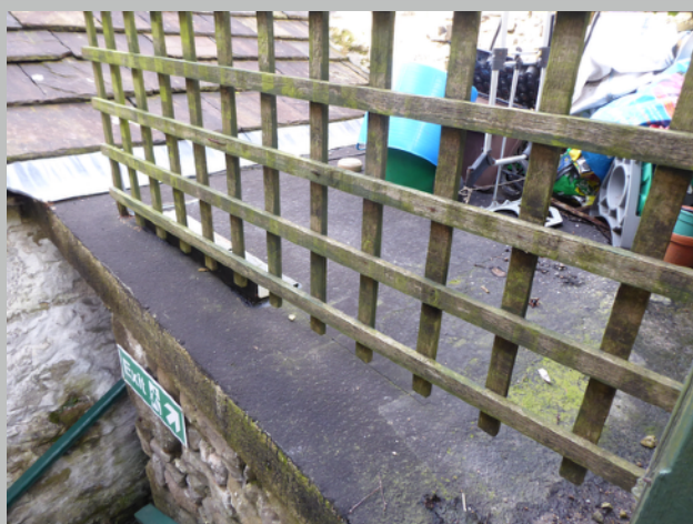
Plate 8. Roof of outhouse
